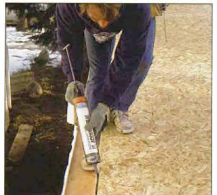
Second-floor rim-joist seal. To provide an air barrier at second-floor rim joists, Tyvek strips are sealed with acoustical caulk to top and bottom wall plates. Here, David Schuman puts a bead of acoustical caulk along the wall before it's raised into place.
