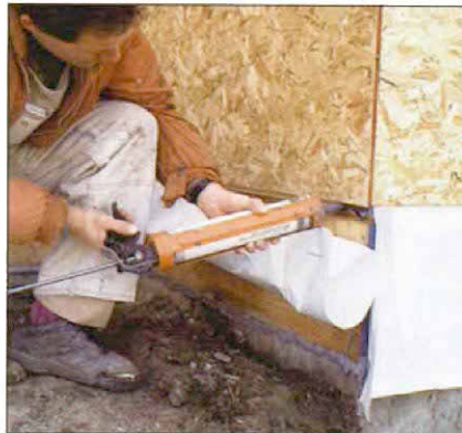
Sealing the rim joist. Builder Peter Amerongen devised an air-barrier technique that uses polyethylene on inside walls and strips of Tyvek housewrap to seal the rim joists. Acoustical caulk seals the top edge of the housewrap to the frame.
